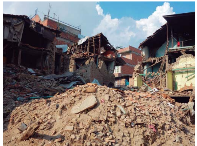
Damage in Nepal from the 2015 earthquake (Photo: JICA)
