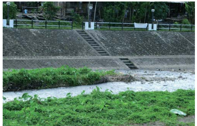
Steps built into the bank protection are used to assess the water level visually during a flood.(Photo: JICA)
